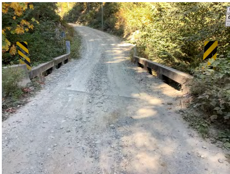
Right Bank Abutment when facing downstream
